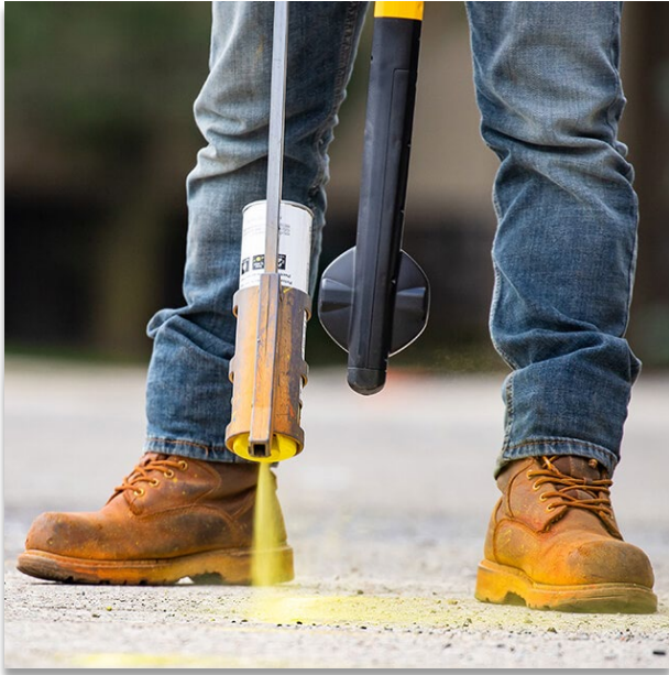
Mark underground infrastructure
