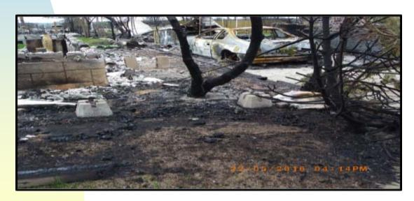
Combustible ground covers allowed fire to spread into contact with homes, while noncombustible ground covers blocked fire pathways
